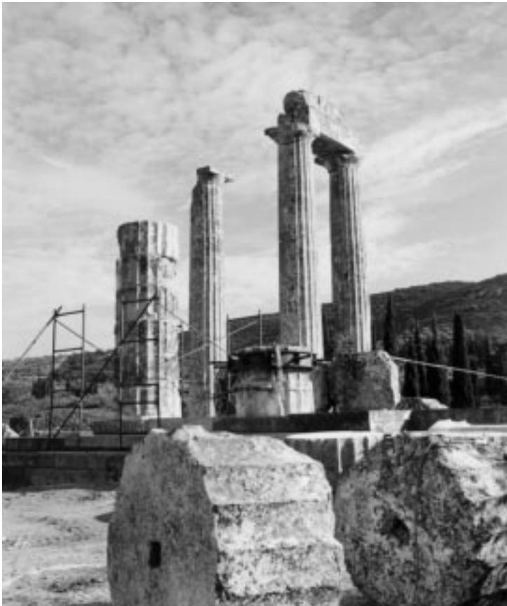
Fig. 16. Two “new” columns going back in place (six drums set on one, two on other, of total 13 in each) on November 29, 1999.
