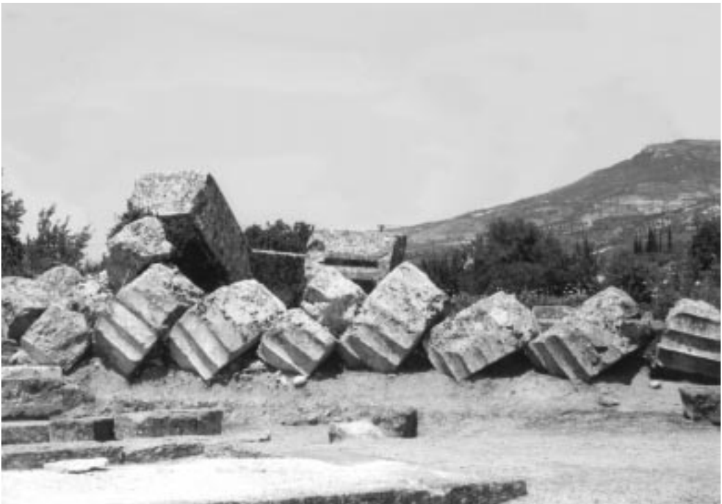
Fig. 9. Fallen drums showing erosion of exposed surfaces in contrast to well-preserved surfaces of lower parts of blocks.
