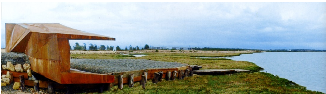
Corten structure at Bahia de Cadiz.
